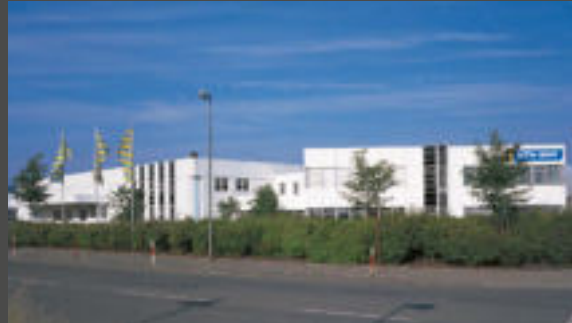
German production facility in Bielefeld
